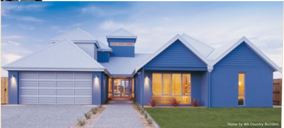
Home by WA Country Builders
